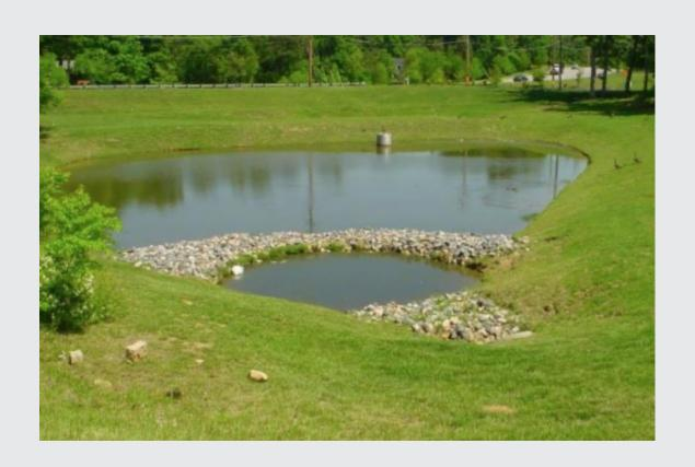
Technique or method designed to manage the quantity and <u>improve the quality of</u> <u>stormwater runoff.</u>
